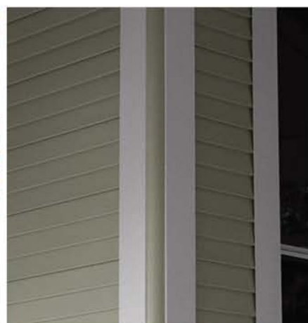
Trimworks® three-piece beaded corner post.
